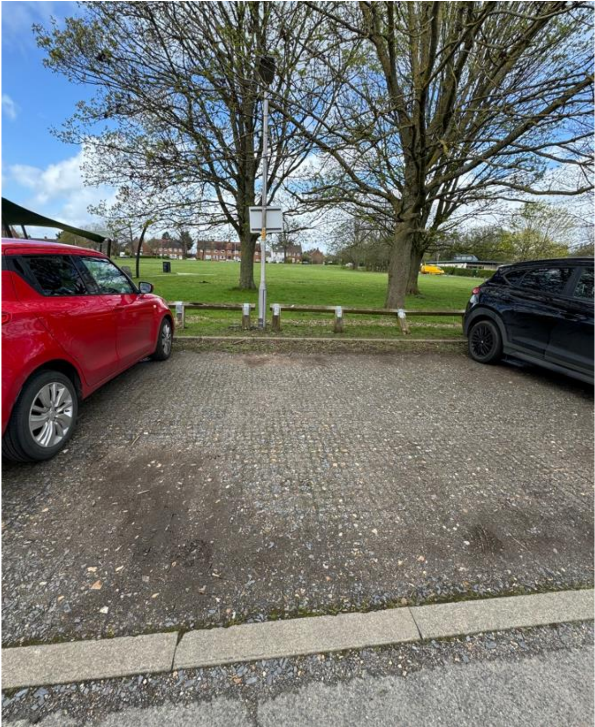
Example of Existing Grasscrete at Southern end of School Mead
